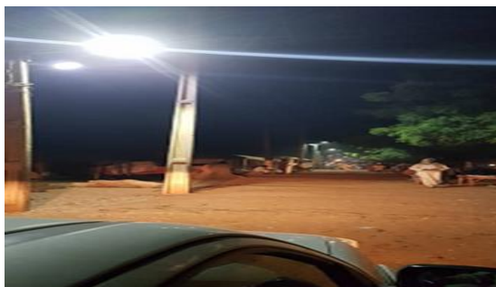
Testing street lights
