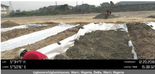
Equipment Foundation Works
