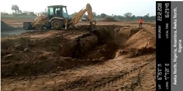
Equipment Foundation Work
