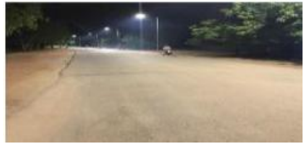
Street Lights Installation Completed
