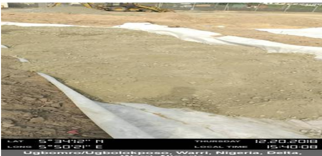
Site Internal Roads Preparations
