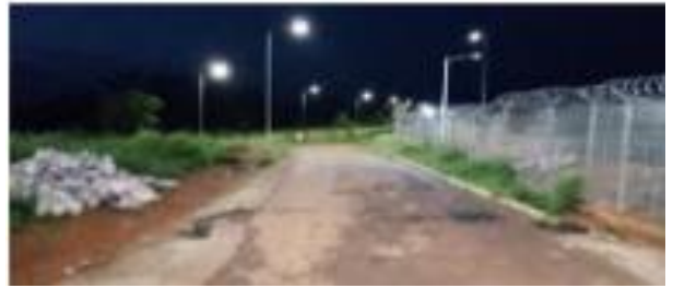
Street Lighting Works Completed
