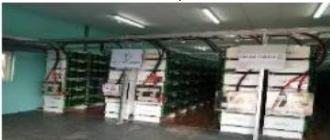
Battery Installed and Commissioned
