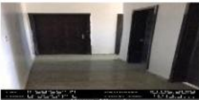
Internal Works of WTC Completed
