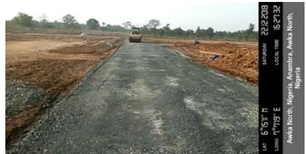
Internal Road Preparation
