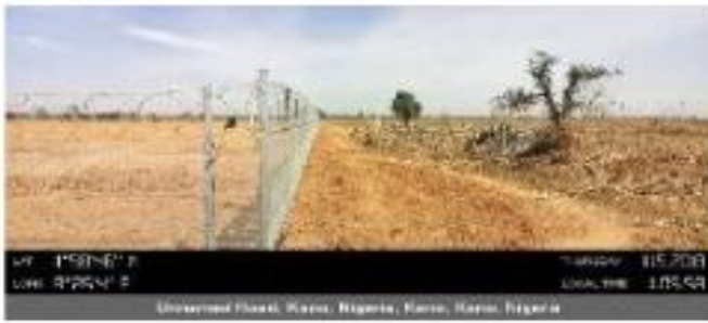
Completed Fencing Works
