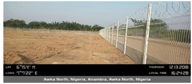
After Site Preparation (Fencing Completed)
