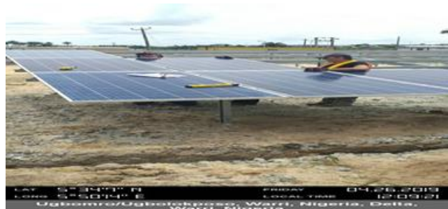
Solar Panels being mounted
