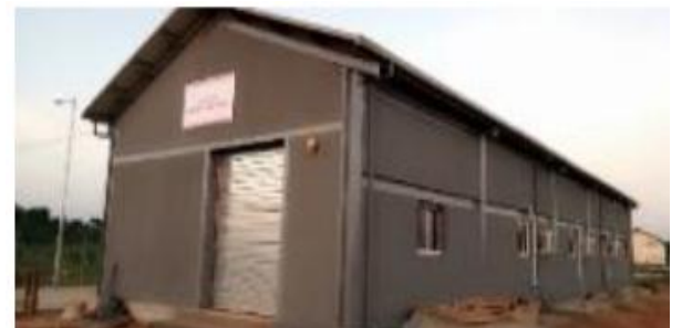
Battery Building Completed
